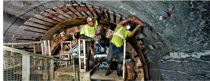
A worker cuts a rock bolt that had secured a weak section of rock from the roof of a train tunnel in New York City, in 2008.
