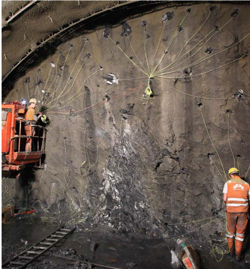
Workers set explosives in May 2014 to create the Brenner Base Tunnel, a train tunnel in Austria.
